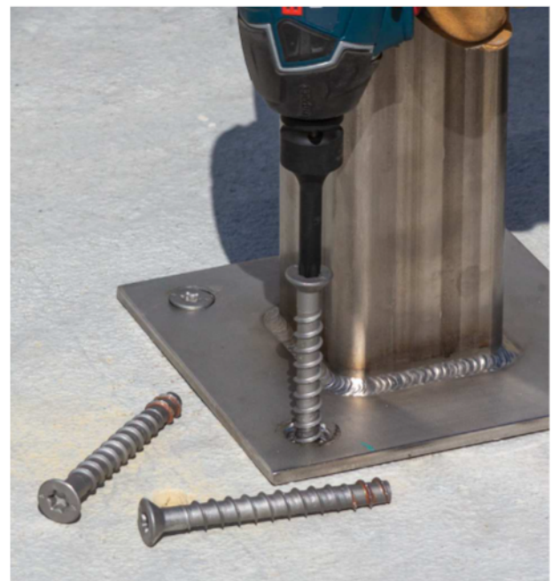
Titen HD Countersunk Installation
