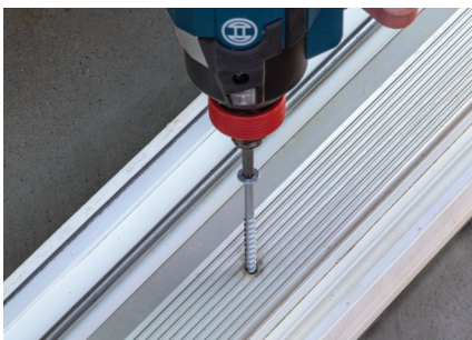
Sliding door track installation
